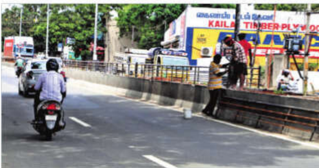
Workers install guardrails on the median along the Pollachi main road at Sundarapuram in Coimbatore on Friday | S SENBAGAPANDIYAN
